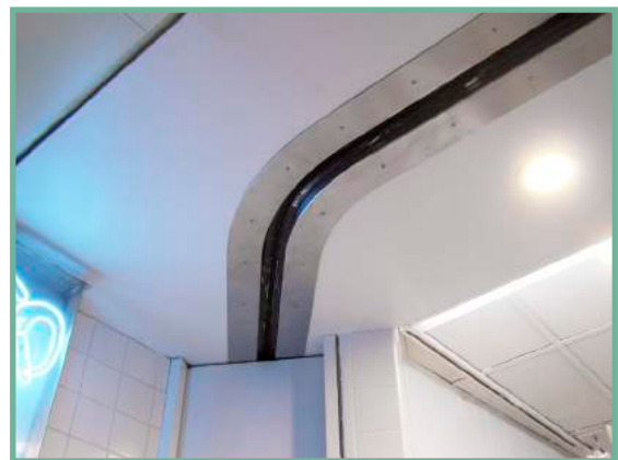
Stainless Steel Track Installed in Auntie Anne's
