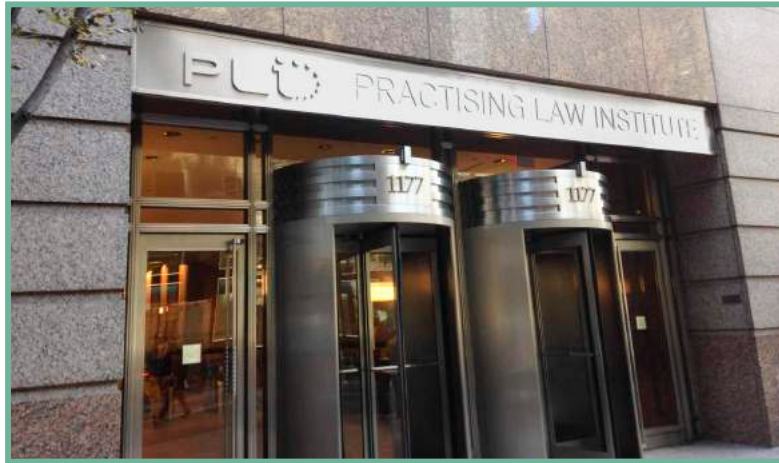
Stainless Steel Panel Modification Installed at Practising Law Institute Located in New York City, NY
